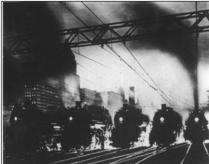
Illinois Central Steam Engines in 1920's Chicago (courtesy of Illinois Central Historical Society)
