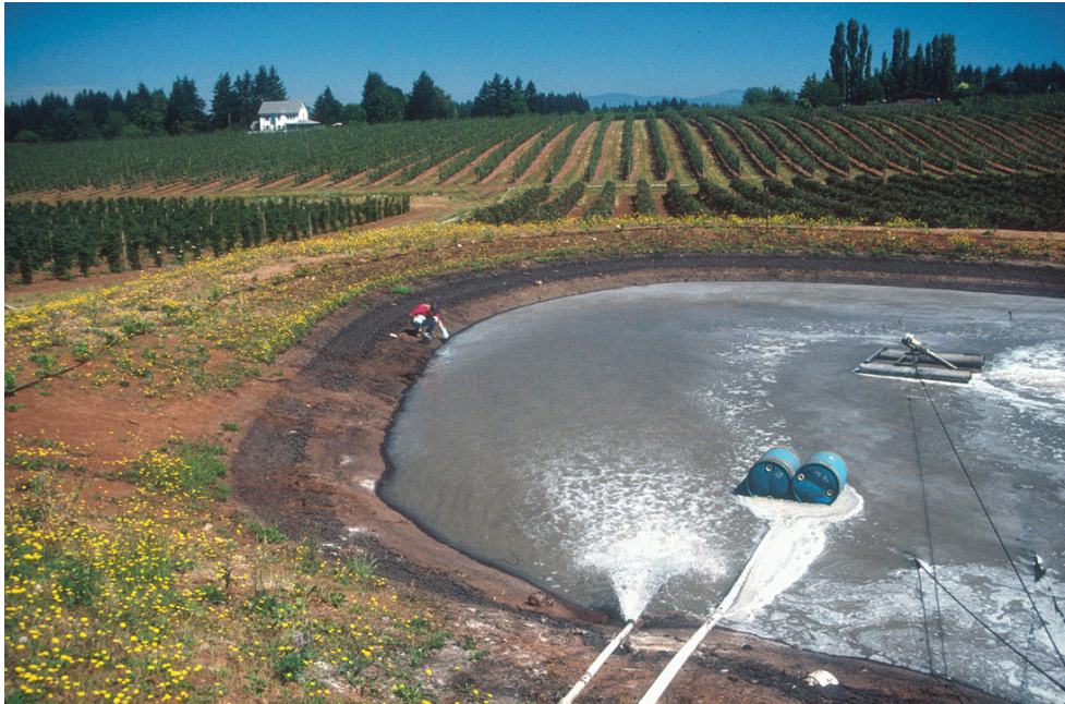
Figure 2-3. Surface impoundment located at a fruit processing facility.
