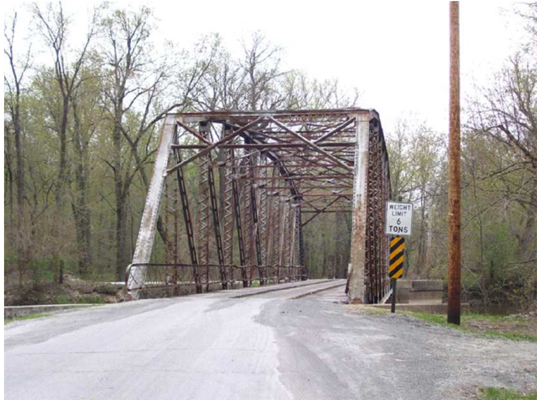
Figure 4.8 County Bridge #36, Range Line Road, Eagle Creek Township, Lake County, Indiana
