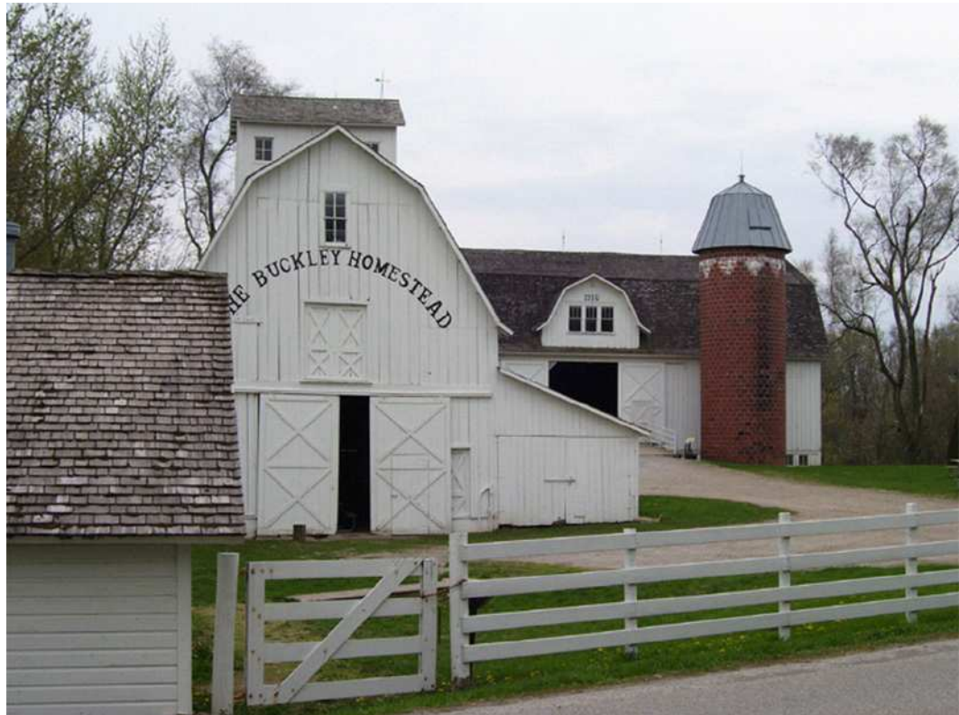
Figure 4.11 Outbuildings, John Buckley Homestead, 3606 W. Belshaw Road, Cedar Creek Township, Lake County, Indiana
