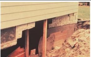
Dry floodproofing is not recommended for keeping surface water out of a basement. The water pressure can break the walls and floor.
