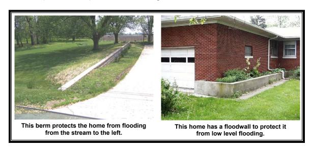
Depending on how porous your ground is, if floodwaters will stay up for more than an hour or two, your barrier will need to handle leaks, seepage of water underneath, and rainwater that falls inside the perimeter. You will need a sump and/or drain to collect the internal groundwater and surface water. A pump and pipe is also needed to pump the internal drainage over the barrier.
