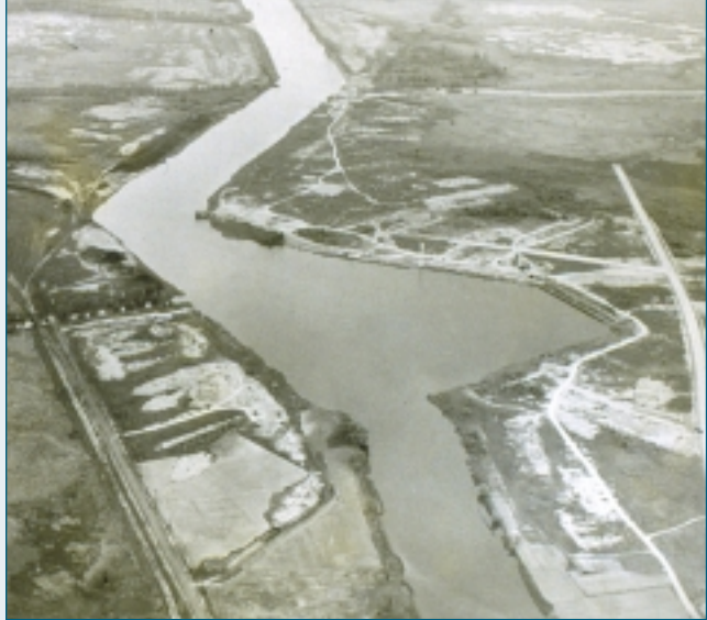
River Raisin with channel straightened and "turning basin" constructed in 1931 to allow for large ships.
