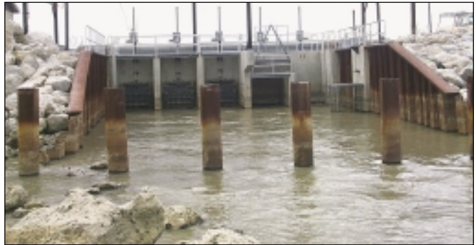
Metzger Marsh. Five large gates provide effective control of the water levels in the marsh, while grates control entry of large fish.
