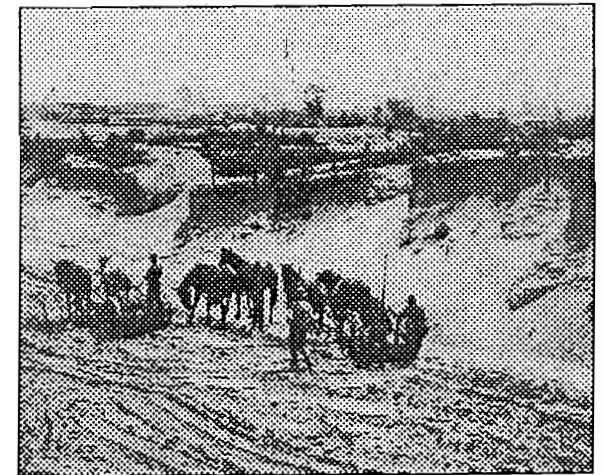
Mule teams excavating the dunes for the Gary Works, 1906.
