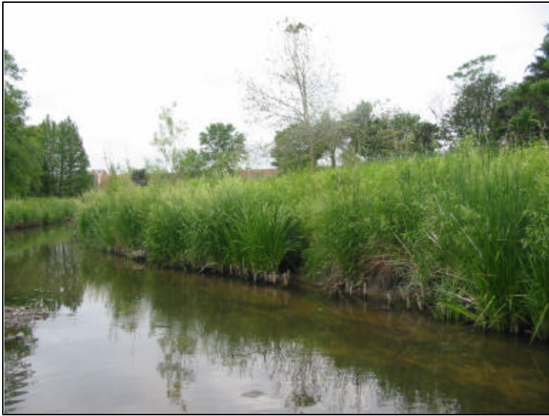
A coir fascine roll on the right bank (installation 7), looking downstream. This coir was in good condition, cord grass and sweet flag were doing well, and stability was very good. Don referred to this as the best wetland/coir log combination seen.
