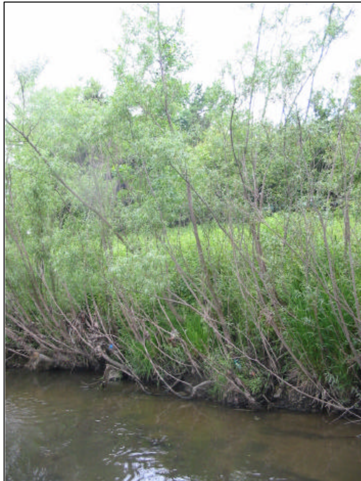
This photo was taken of the willow stakes on the right bank (installation 6). This is the most successful example of willow installation.
