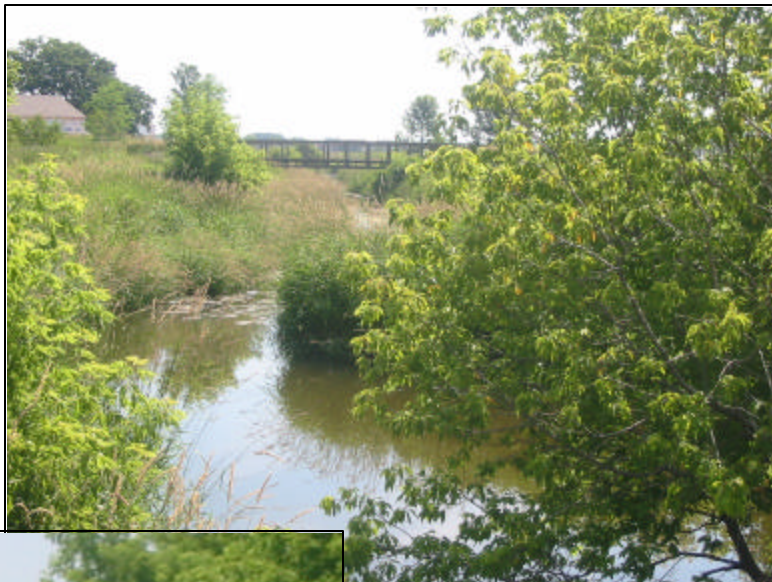
Looking downstream from the footbridge
