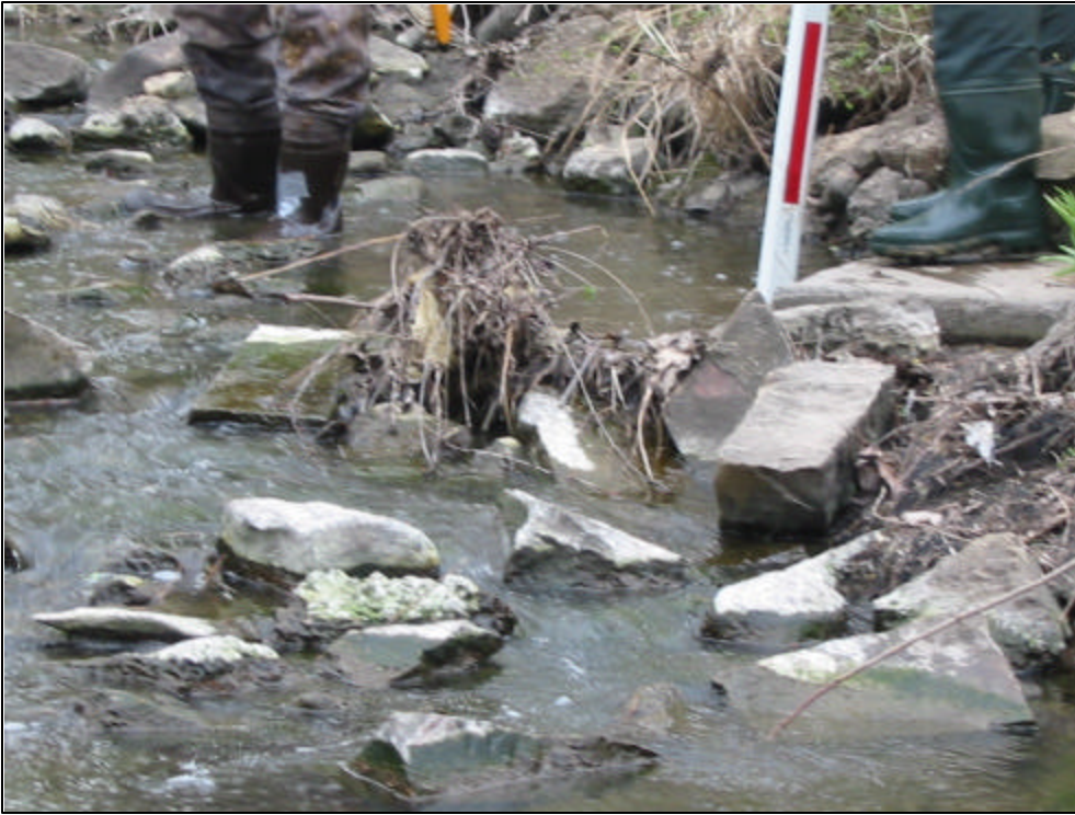
Remnants of vortex weir:
