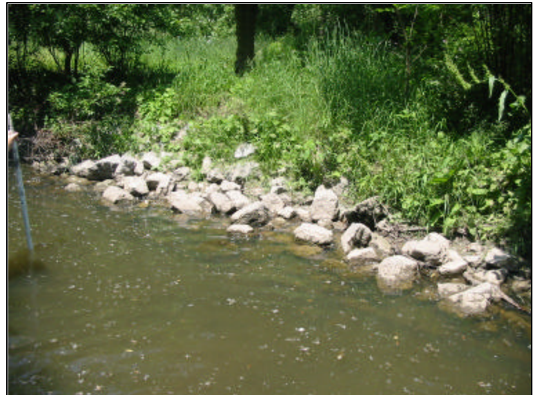
Buried lunkers covered with rock upstream of the fourth Newbury weir. Lunkers were open to a depth of about 1 foot. There was some erosion resulting from the lunkers being put in too deep.
