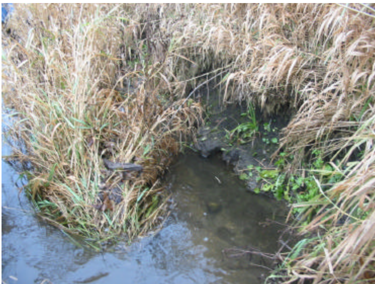
25 feet of severe slumping on the right bank just downstream of the riffle pictured above.
