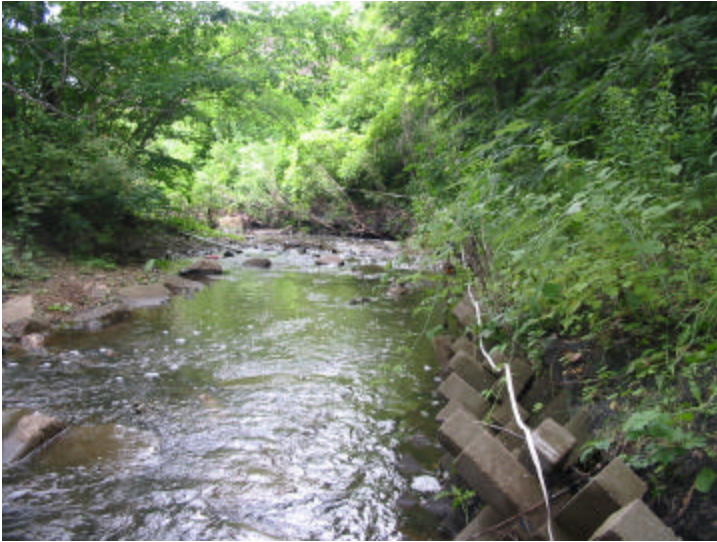
Looking downstream at the ajacks and geogrid that make up installation 1 on the right bank.
