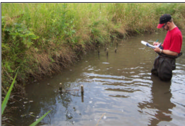
The biolog washout on the right bank at installation 6. Note the stakes with nothing behind them.
