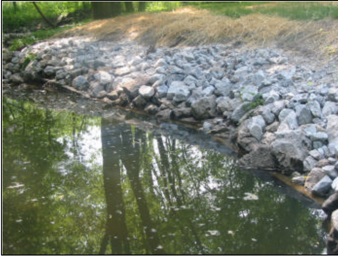
Wooden lunkers on the right bank covered with rock on North Branch channel. At the upstream end the lunkers were halfway filled with sediment; farther downstream the lunkers were more open. The native plantings above the lunkers appear to have been trampled.
