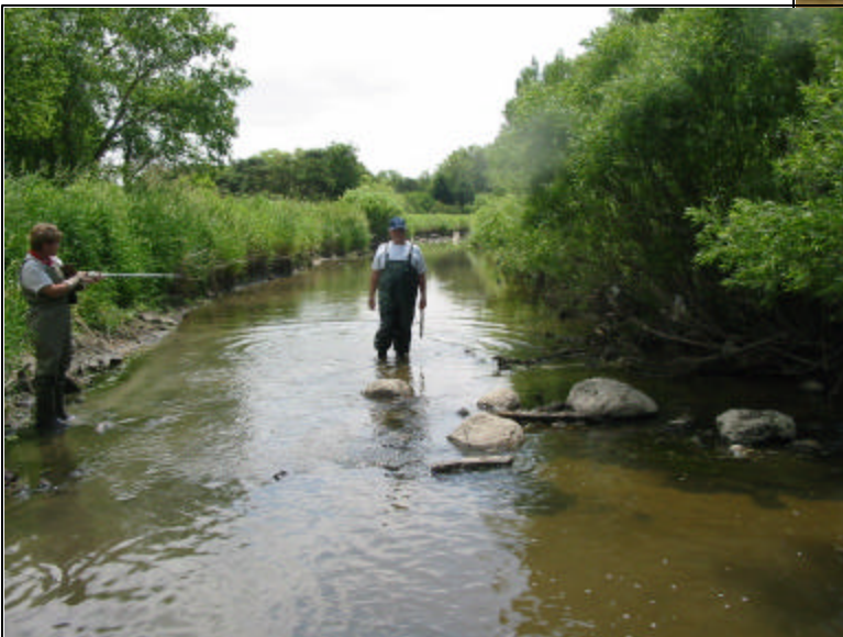
An inverted vortex weir (part of installation 9). Notice the rocks which have moved out of position.
