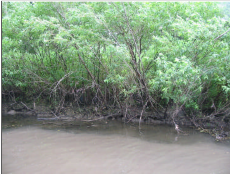
Broad view of the brush layer and willow stakes on the left bank (installation 2). Willow survival was good.
