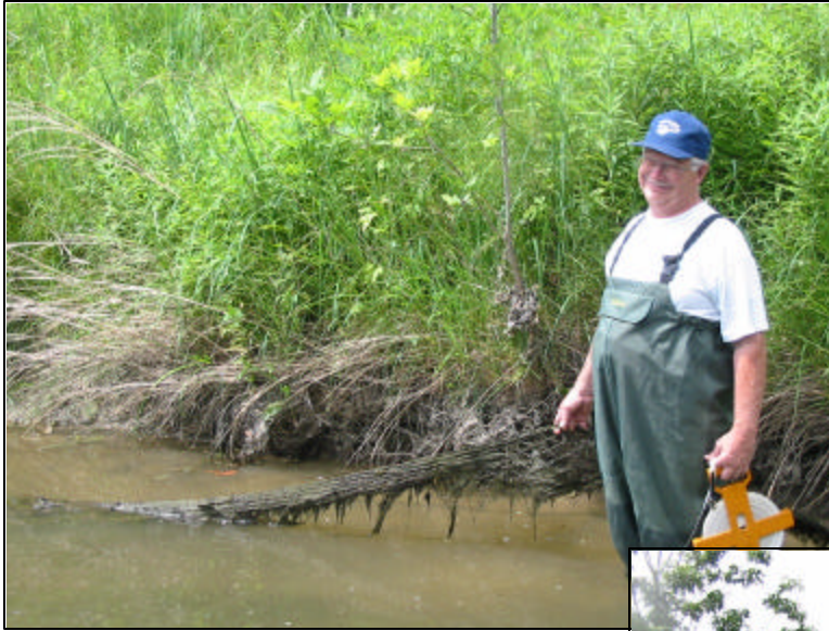
A biologist planted offshore (right bank) with water behind it – the coir fascine is empty (installation 8). This was the most eroded section.
