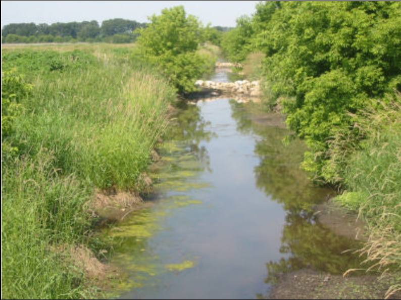
Looking upstream from the footbridge at the riffle installations. There is 155' between the first and second riffle and 165' between the second and third.
