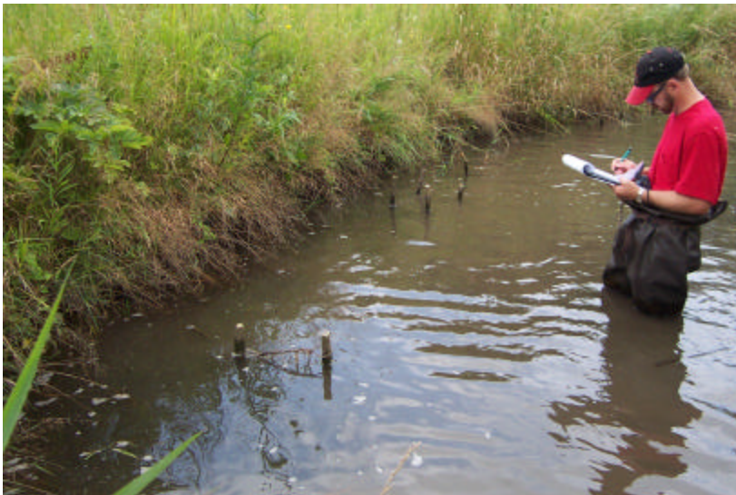
The fiber rolls originally held in place by these wooden stakes are missing
