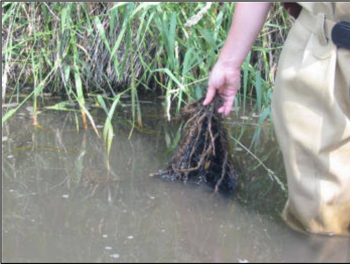
Laura holding up a part of the biolog on the left bank which was submerged under water at the upper end of the biolog installation.
