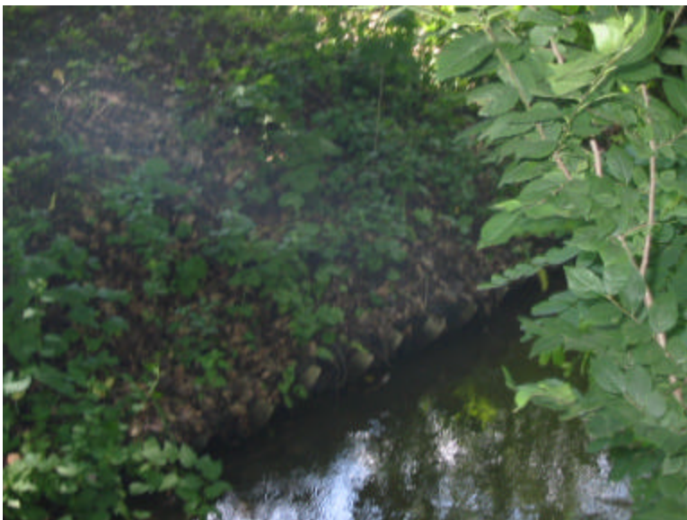
A view from the left bank of the ajacks and fabric of installation 3
