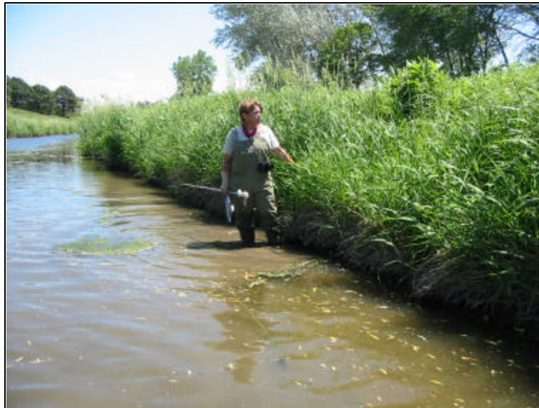
View of a very successful coir fascine installation (installation 19).
