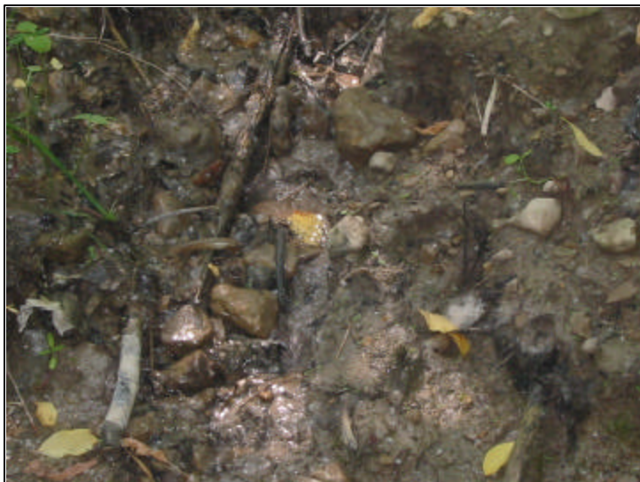
This photo was taken of a sliding seep area between the first and second weirs. The series of weirs installed along the southern channel were designed to reduce energy and sliding. A rebar was originally installed here to measure sliding, but was missing on the day of the site visit.
