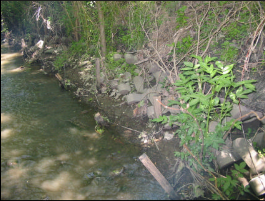
Closer view of ajacks embedded in the toe. Substrate is very soft, with material ranging from silt to small gravel.
