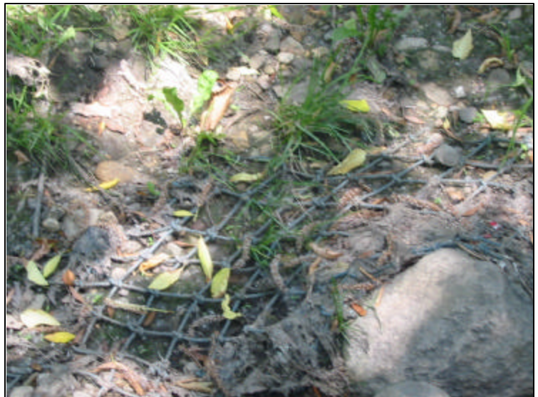
The remains of a biolog put in to stabilize the bank since the weir was not keyed into the bank.
