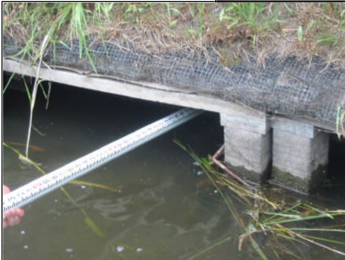
The lunkers were open to a depth of about 1.2 feet
