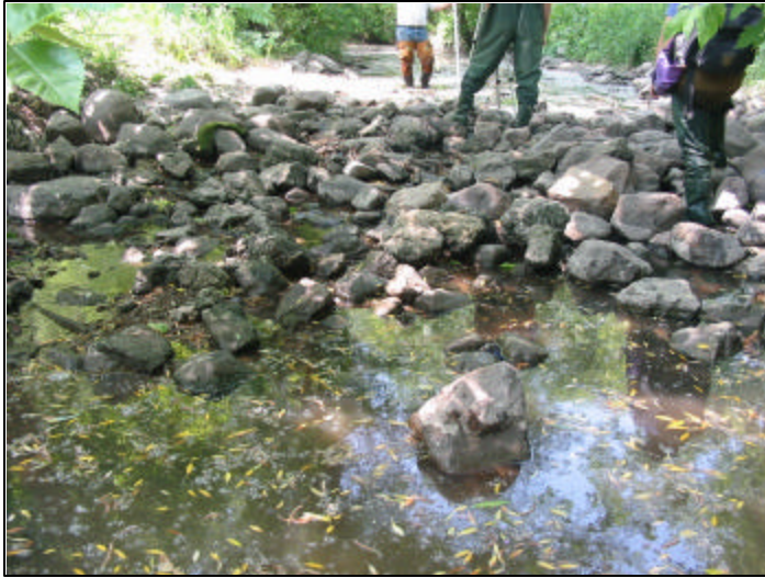
Newberry weir near the north end of the southern channel. This weir is raised up to direct water into the forebay of the created wetland; the weir is not keyed into the bank and it appears to have stabilized the instream area.
