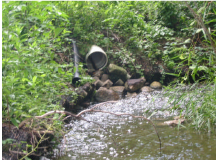
18 inch culvert inlet pipe on the outside bend of the right bank (installation 3). Ajacks and fabric can also be seen here.
