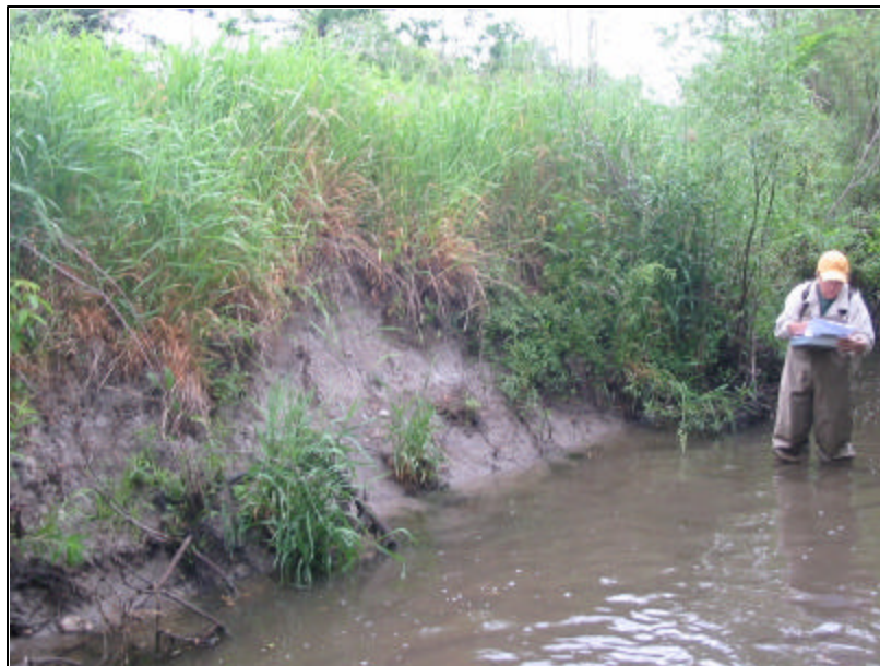
Scour on the right bank between installations 1 (willow stakes) and 2 (brush layer with willow stakes).
