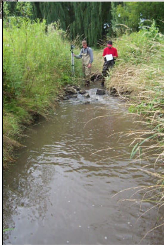
This photo was taken of riffle 3 where pool depth was 0.8'-1.0', the substrate was cobble and artificial large rock, and planting survival was good.
