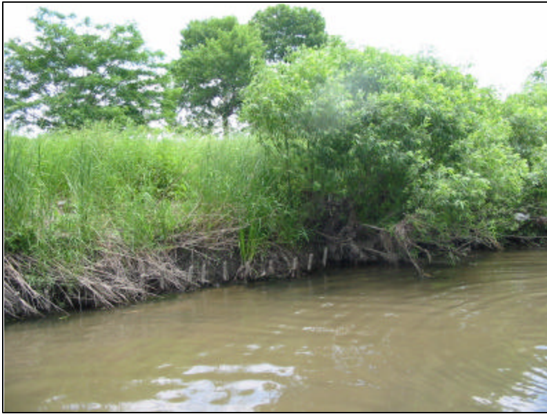
The left bank and coir fascine with cord grass at installation 10. Planting survival is good here.
