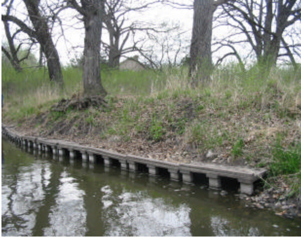
Lunkers installed high on the bank
