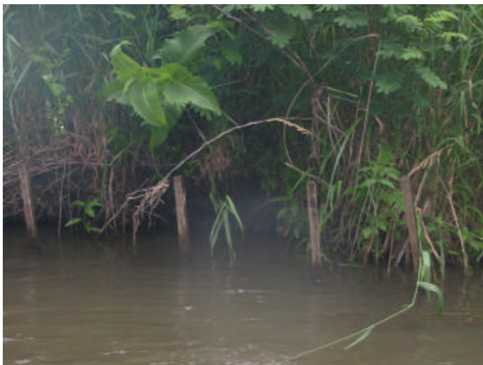
Stakes at installation 8, which is made up of 175' of fiber rolls and stakes. The pool depth varies a lot along this practice and the "islands" pictured above have formed in the channel. Pool depth was 3.5' at the upstream end of this practice.
