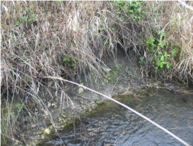
Close up of a slumping, undercut bank near the upstream end of the project where the gradient was steep and stability was not very good. Buffer species were dominated by reed canary grass.
