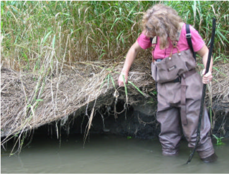
At installation 4, where bank grading and fabric were installed, 2 rolls of fabric were found, one overlaying the other. In some areas the bank was eroded and undercut behind the fabric.
