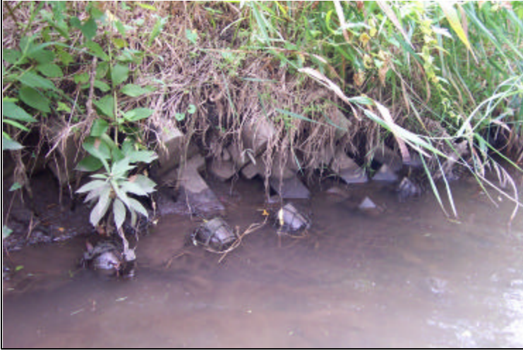
The ajacks at the upstream end of the site (part of installation 1).
