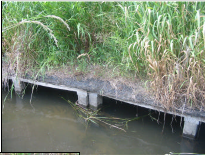
View of the lunkers and mattress (the fabric above the lunkers).
