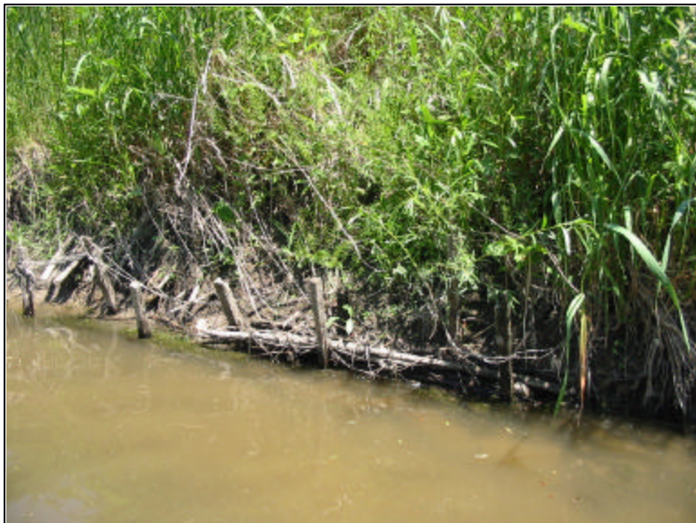
A close-up photo of the brush fascine (installation 13).
