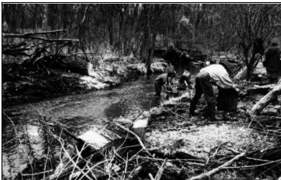
Exhibit 401a: Logjam Removal Using Hand-Held Tools (Source: CBBEL Files)
