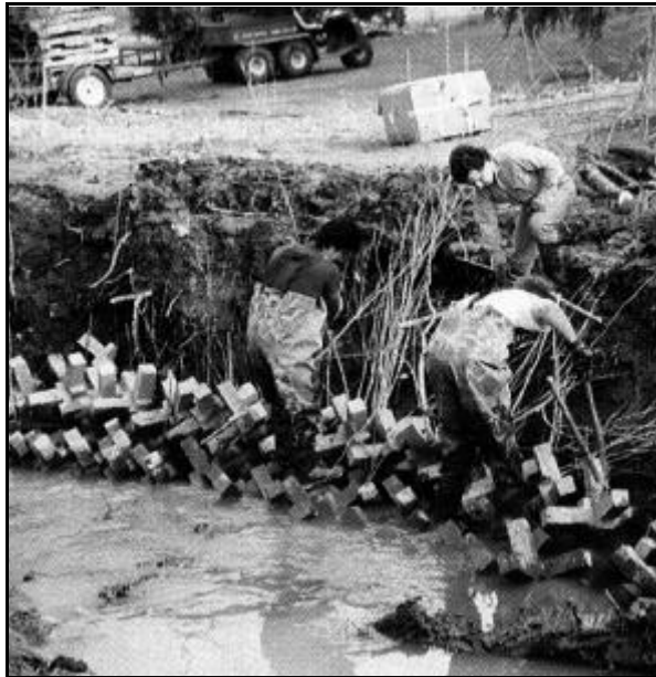
Exhibit 509a: A-Jacks Installation (Source: Illinois State Water Survey Publication)
