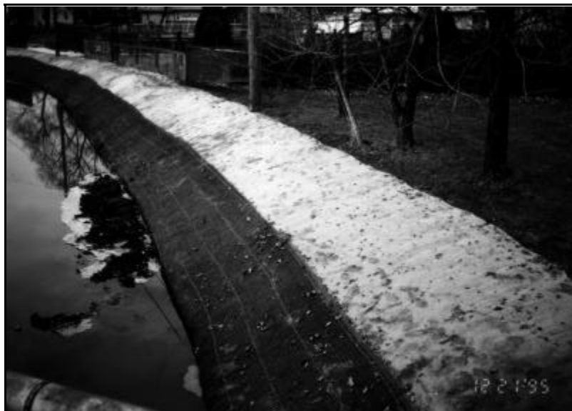
Exhibit 1104a: Erosion Control Blanket (Source: CBBEL Files)
