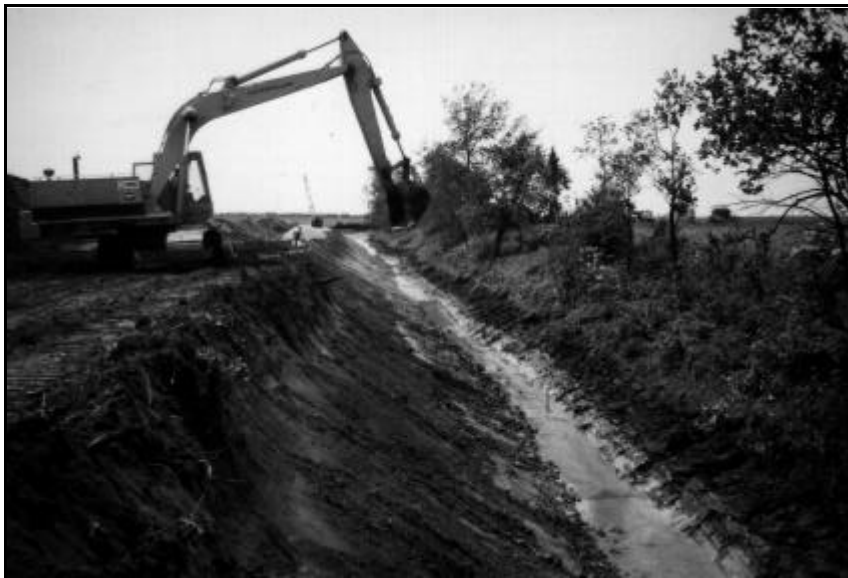
Exhibit 602a: Channel Excavation/Dredging (Source: NRCS Files)
