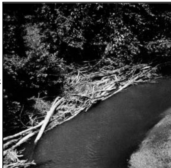
Exhibit 403f: Anchored brush piles are an inexpensive but effective means of bank protection (Source: Ohio Stream Management Guide)
