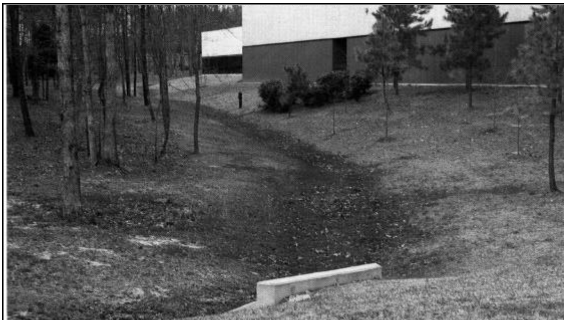
Exhibit 701a: Channel with Grass Lining (Source: North Carolina Erosion Control Manual)
