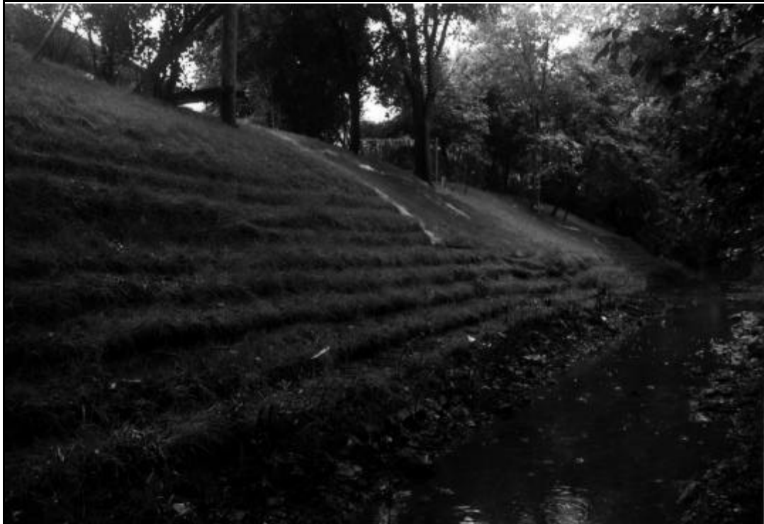
Exhibit 506a: Vegetative Geogrid (Source: Biotechnical Erosion Control Limited)
