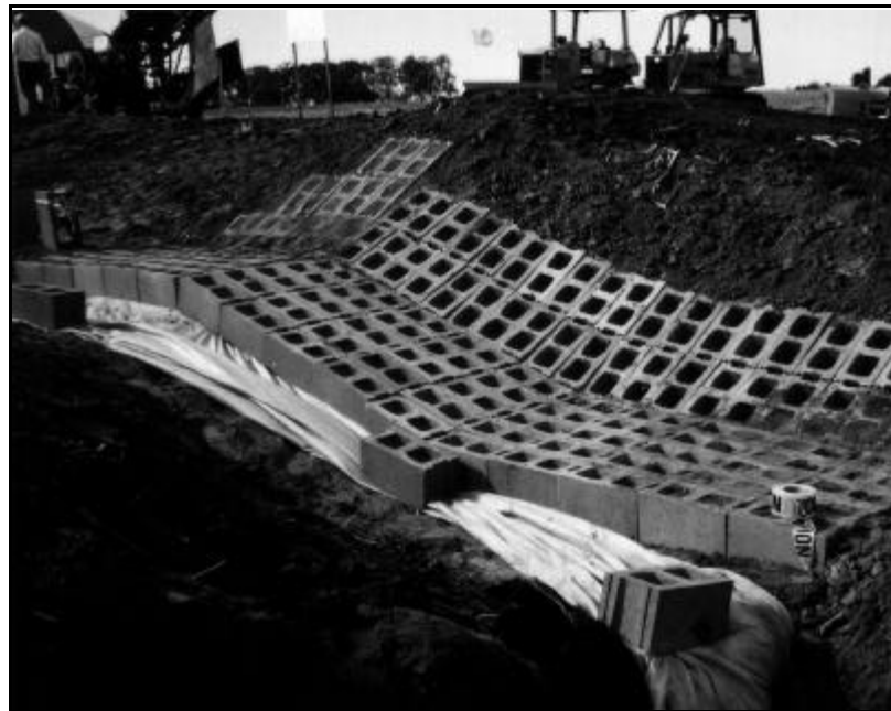
Exhibit 705c: Concrete Block Chute (Source: CBBEL Files)
