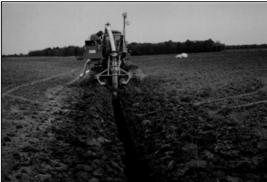
Exhibit 201a: Tile Drain Installation (Source: NRCS Files)
