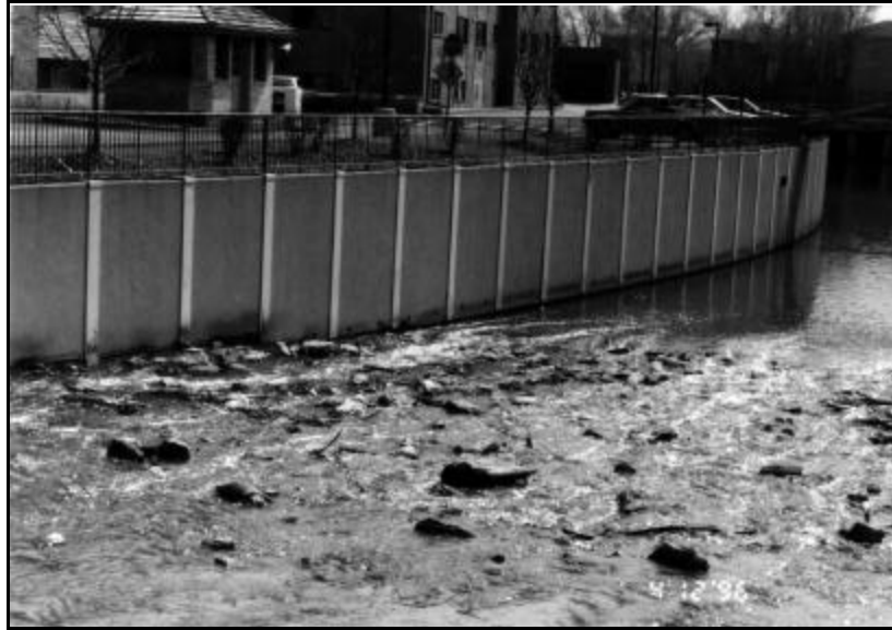
Exhibit 515a: Composite Retaining Wall (Source: CBBEL Files)
