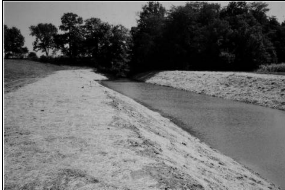
Exhibit 801a: In-Channel Sediment Basin (Source: NRCS Files)
