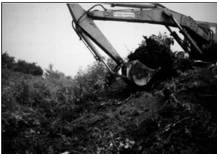
Exhibit 107a: Clearing and Grubbing (Source: NRCS Files)
