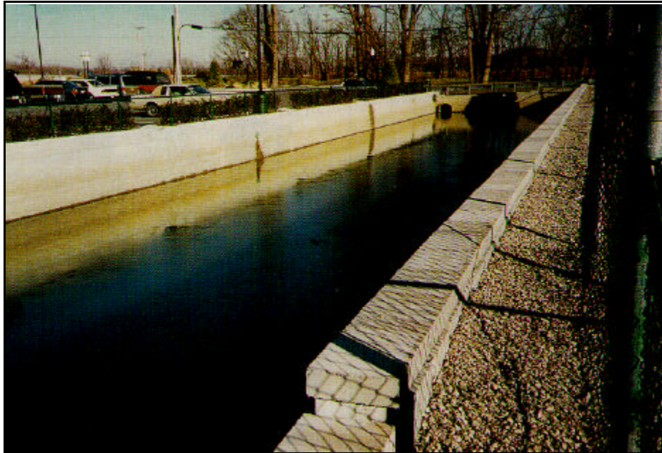
Exhibit 511a: Concrete Retaining Wall (Source: Land and Water Magazine)
