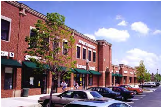
This newer building is broken down into a series of storefronts to address a pedestrian scale.
