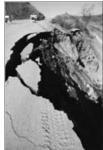
Subsidence, slippage, and other kinds of slope failure can damage structures.
