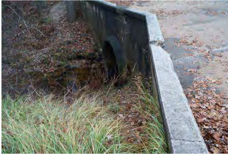
Figure 33. Daylighting in Dunes Creek (2005)
