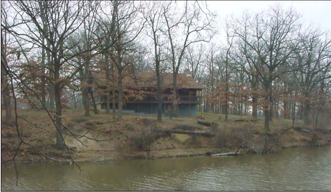
Figure 6-6: Shoreline Erosion at Jerry Pavese Park
