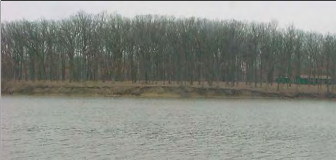
Figure 6-8: Shoreline Erosion at Fred Rose Park
