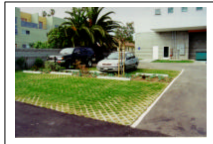
Figure 7, 8. On left, biofilter/swale system in parking lot of a school receives all runoff. For almost all storms, all runoff remains onsite for infiltration. On right, permeable pavers in a parking lot of a business allows runoff to infiltrate instead of run off into the street.
