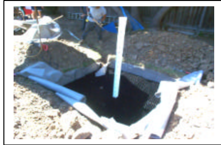
Figures 5, 6. Use of plastic in-fill instead of gravel allows greater storage volume, 94% versus 40%. On left, sub-surface infiltration trench filled with RainStore ; on right, trench filled with StormCell .
