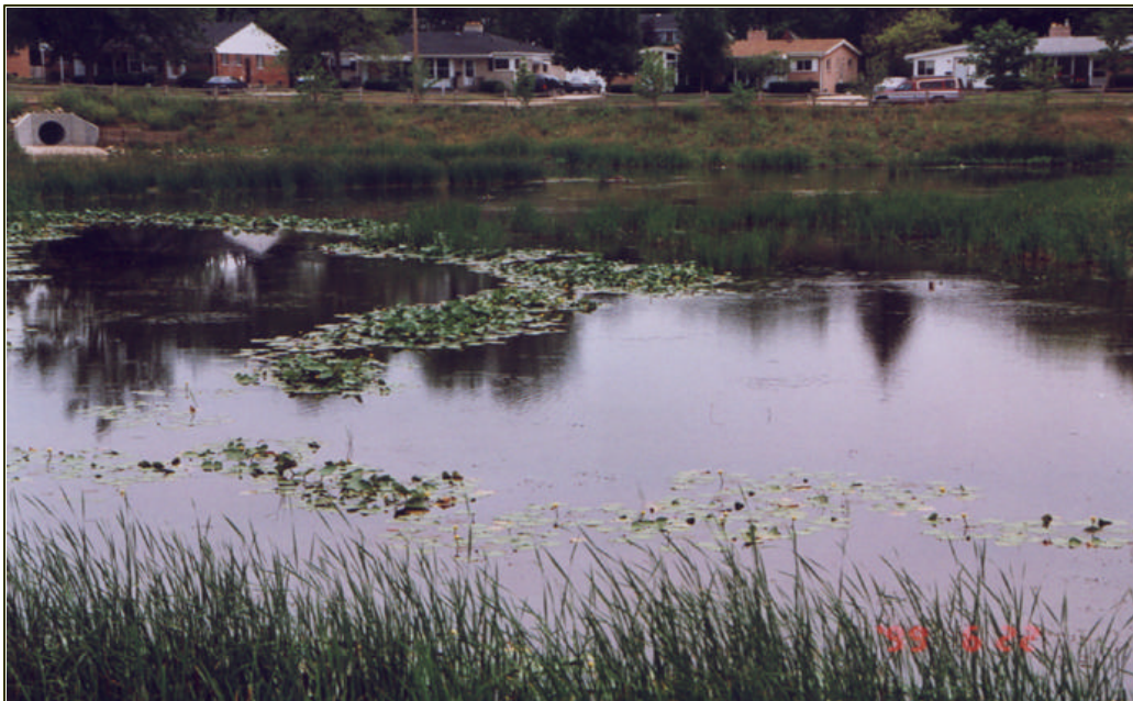
Figure 4 -Example of constructed wetland -- Tollgate Storm water Treatment Facility Lansing, Michigan (courtesy of Patrick Lindemann, Ingham County Drain Commissioner, and designer of the project)
