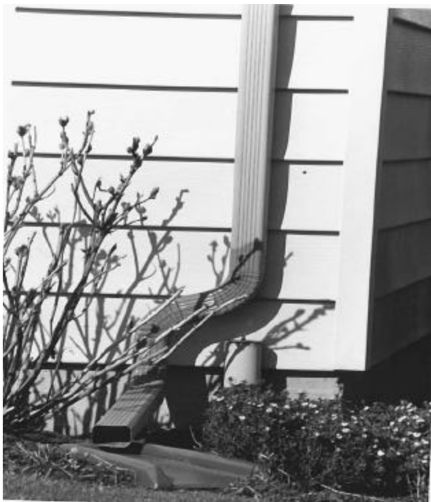
(Figure No. 3) Typical Residential Downspout Disconnection
