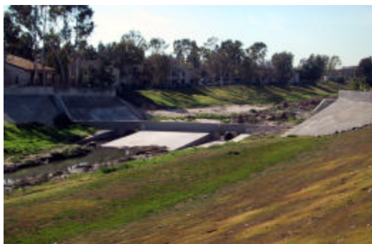
Photo 1 & 2 - San Diego Crk, looking downstream at grade control structure between East Yale Loop and Creek Rd.
