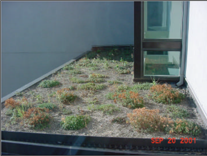
Figure 15. Buckman Terrace EcoRoof at the building entry with protection from north facing wall
