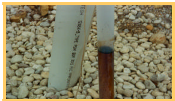
The plastic bailer on the right shows free product floating on top of contaminated groundwater. Bailers are used to collect groundwater samples from monitoring wells.
