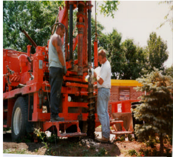
Workers drill a boring to collect soil samples.
