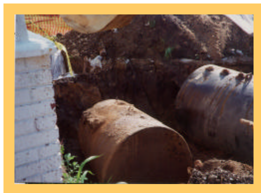
The proximity of the white brick building has complicated tank removal.
