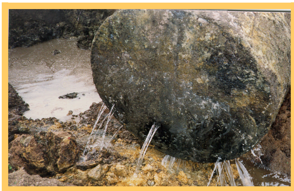
This excavated tank shows how a few small leaks can cause a big problem.
