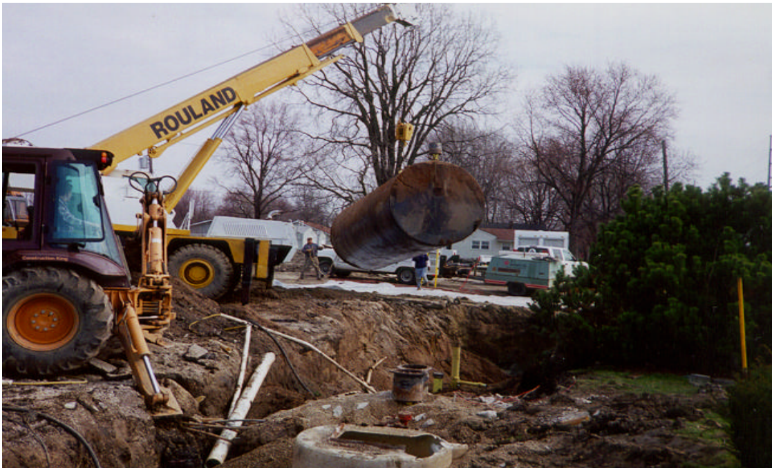
UST contractors remove a tank.
