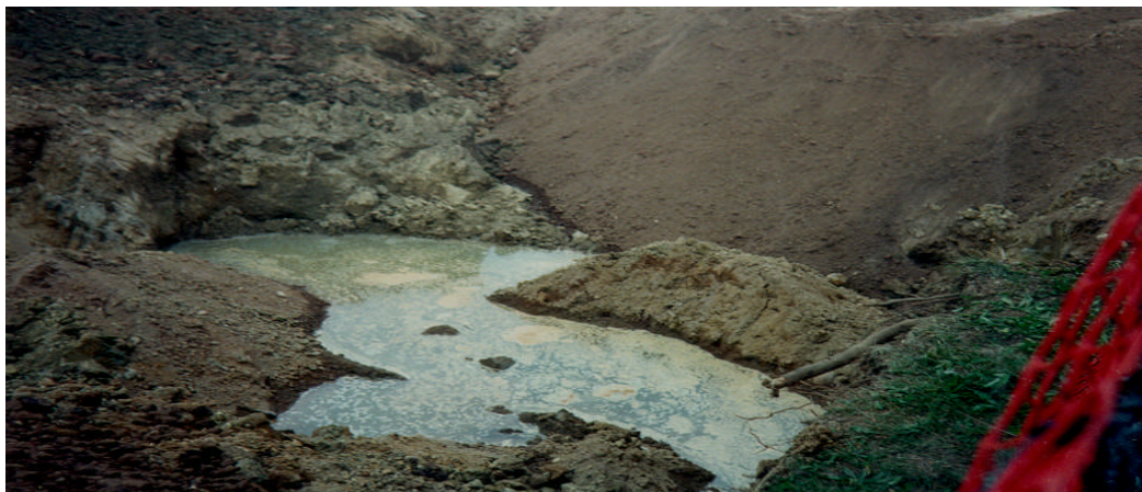
Groundwater in this tank excavation pit shows a petroleum sheen.
