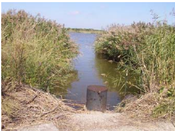
Figure 33: Structure #15, facing North (Conservation Area Outlet)
