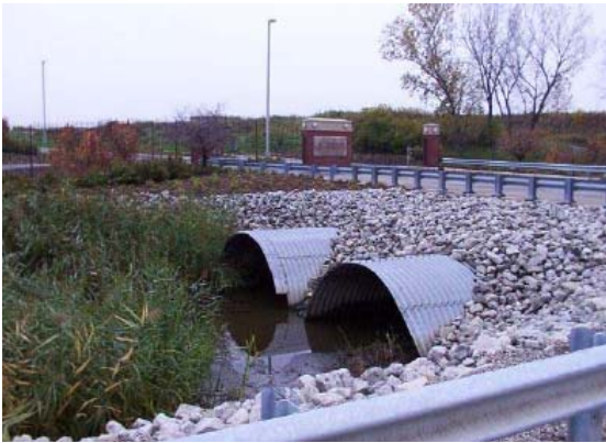
Figure 38: Pullman Creek Channel facing upstream
