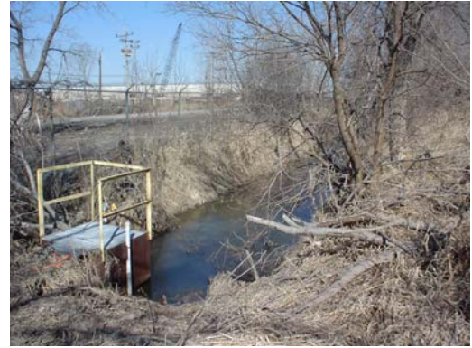
Figure 28: Structure #1, facing North
